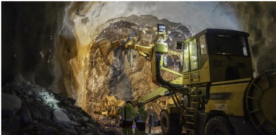
Drilling for bolting. courtesy of Nils Janestad
