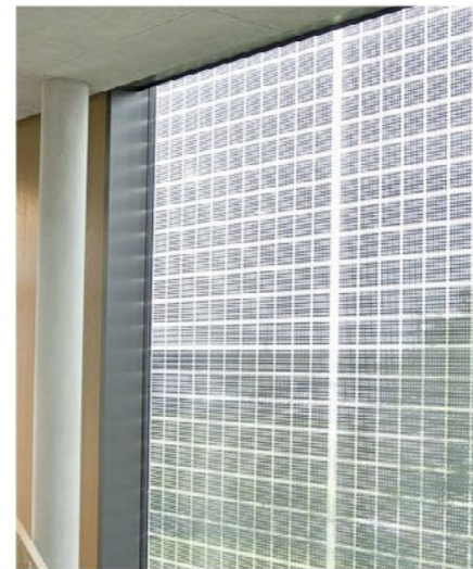
Solar cells on glass Source: resources.made-in-china.com
