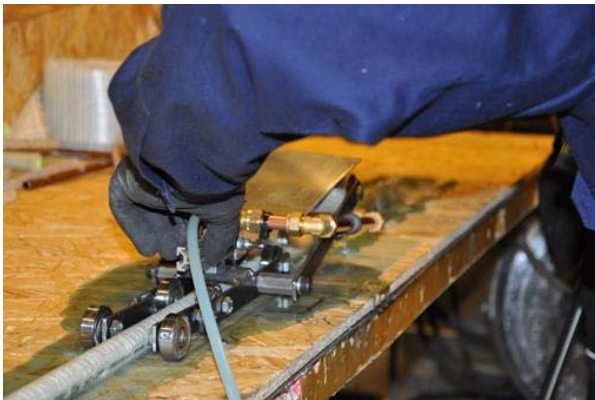
Figure 23 Development of equipment for attaching a tube in narrow spaces.
