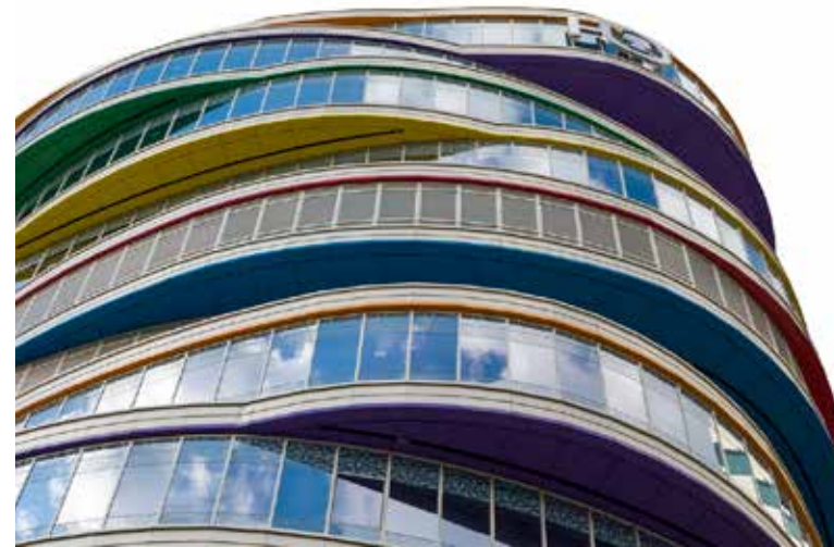
THE BUERGER CENTER The organic building
