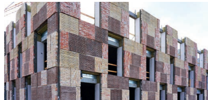
REUSED MATERIALS - From demolished buildings on site.
