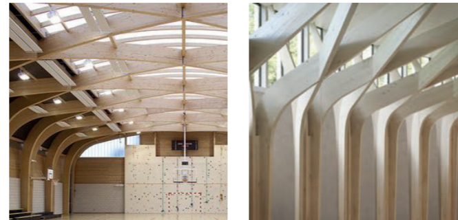
ARCHES - Laminated wood to highlight entrances.
