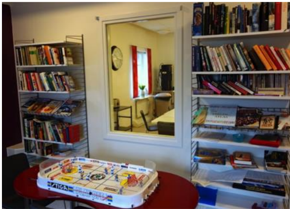
Figure 19. Observation window between two communal rooms in a SiS facility for adult males. The break-resistant glass blocks noise travel between the spaces. The window enables staff in one room to observe a large portion of the other, but might permit residents to conceal themselves in room corners. (Photo by R. Ulrich)
