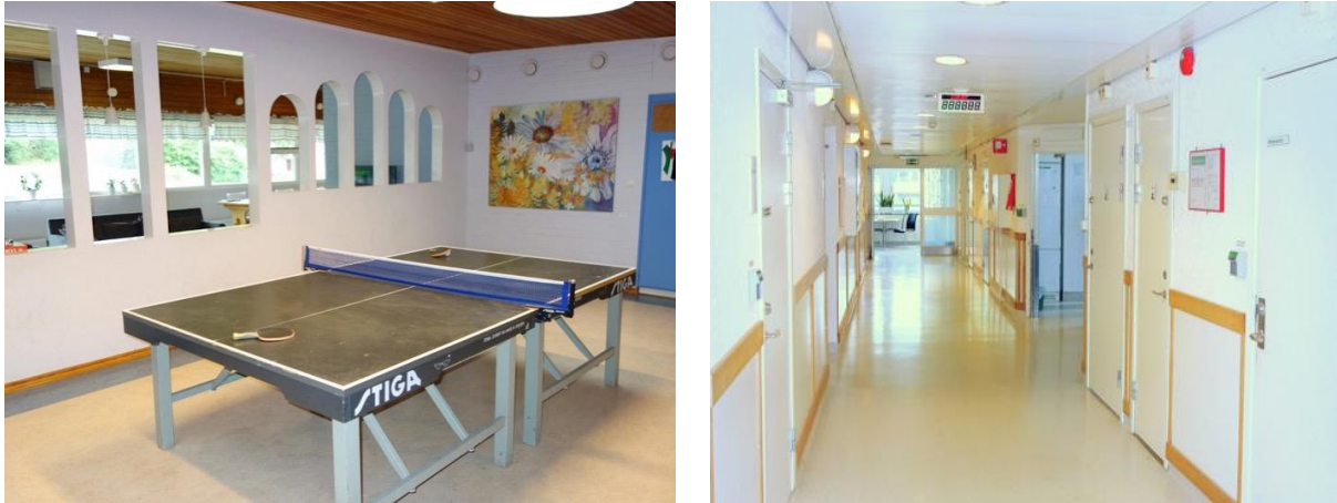
Figure 20. A game room in a SiS youth living unit. Several window-like wall openings enable staff to observe the game room from the adjacent living room, and vice-versa. However, the unglazed observation openings enable noise to propagate throughout both large rooms. (Photo by R. Ulrich)
