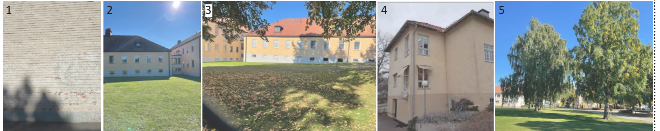
1 The buildings in the area have painted or slammed yellow walls with red brick underneath
