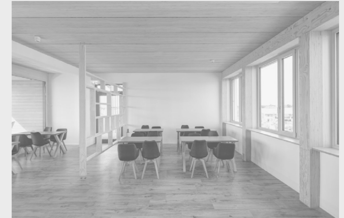
Timber skeleton structure: Steico headquarter, Feldkirchen, Germany
