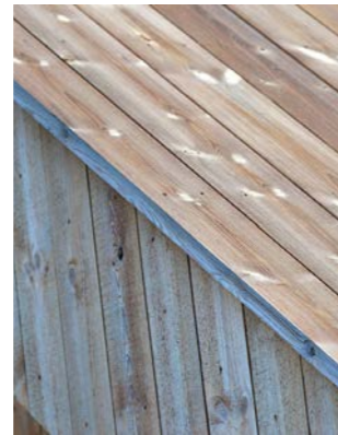
Wooden roof cladding
