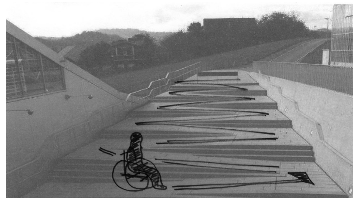
COMBINED RAMP AND STAIRS
