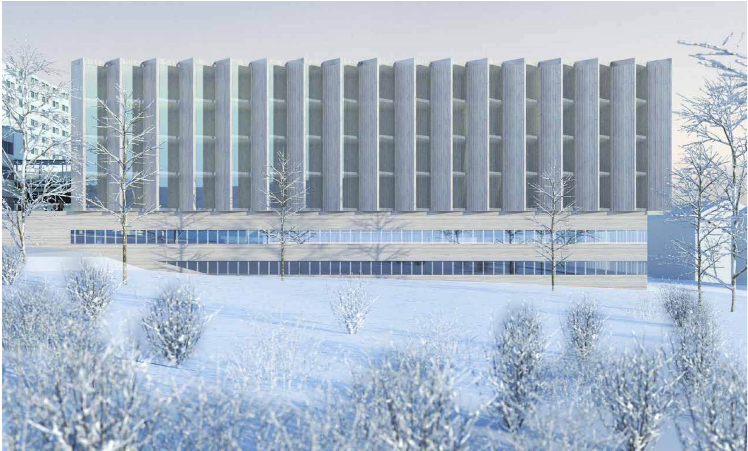
Exterior ward building - north facade
