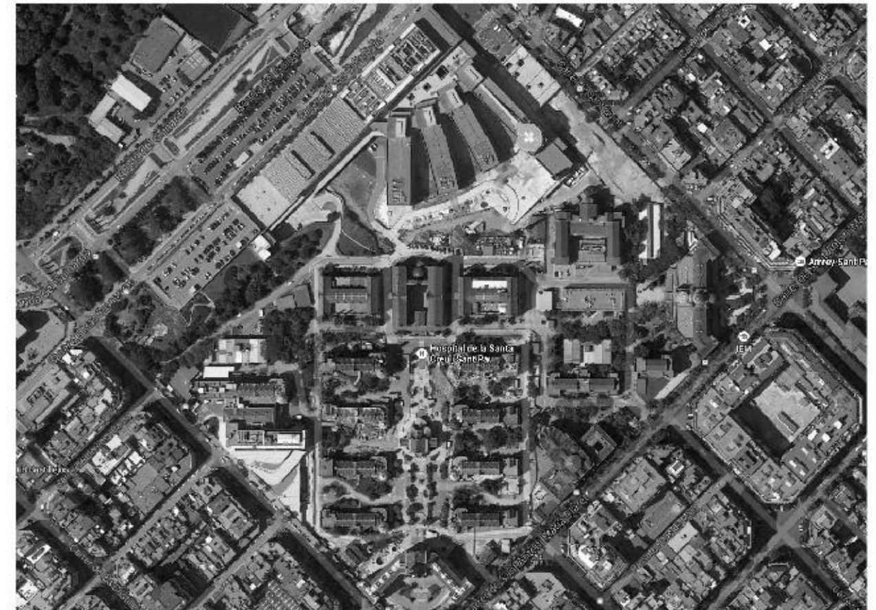
Hospital De la Santa Creu i Sant Paul, Barcelona. New(top) and old hospital parts and spaces between them, can be easily compared.
